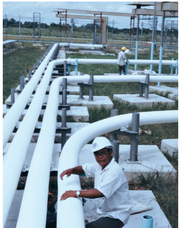
RFS 9-inch cable installed for BBC World Service in Thailand
