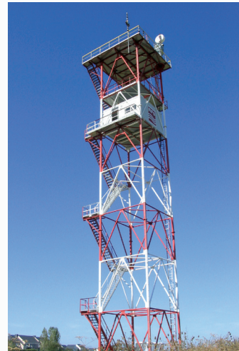
Test range for large antennas
