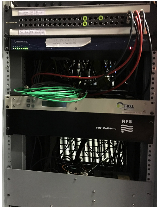
An RFS BAS IMF fully integrated in a rack.
