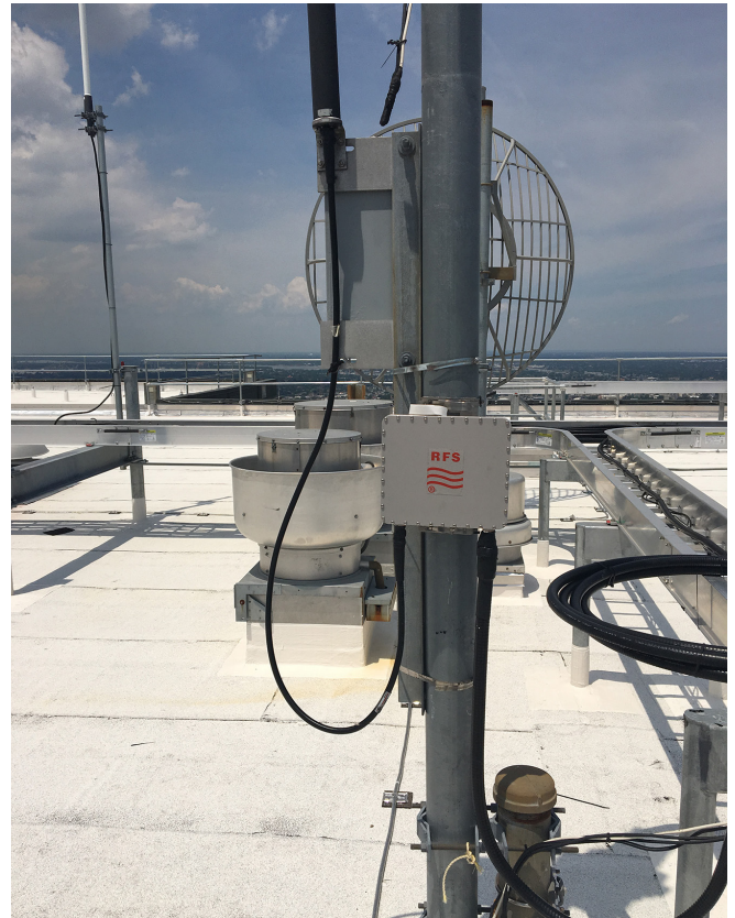
A BAS Interference Mitigation Filter installed in a rooftop setting.
